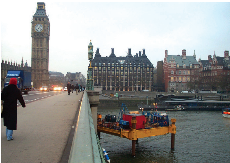
Marine Example: Intrusive survey from a jack-up barge on Westminster Bridge, London
